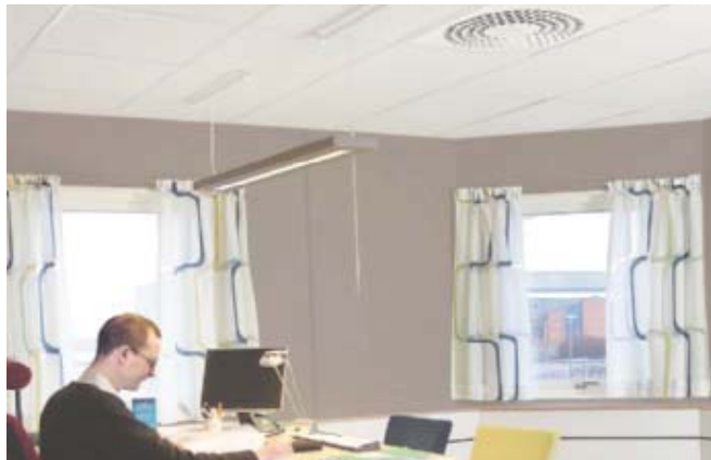
FIGURE 20. A ceiling mounted supply ATD in an office environment.
