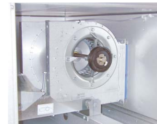
FIGURE 2. A double-inlet radial fan.
