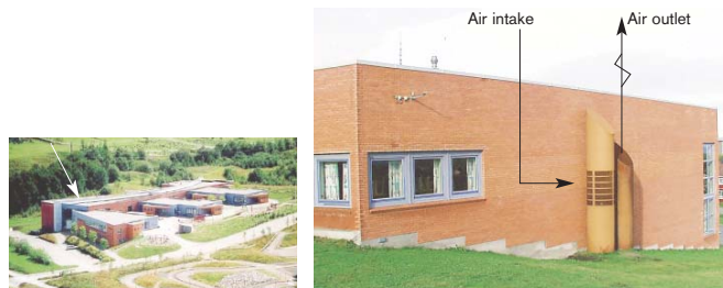
FIGURE 2. Left, a primary school in Trondheim, Norway situated on a hill on the edge of the town close to vegetation and trees. Right, the outdoor air intake and the exhaust air outlet. Rain and snow falling on the intake can be easily sucked into the ventilation system. Photo: Olav Struksnes, Project thesis 2002, EPT-NTNU.
