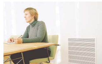
FIGURE 43. A diffuser built into a wall.
