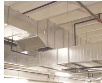
FIGURE 5. Transverse-stiffened duct.
