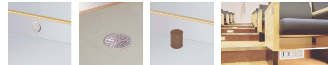
FIGURE 44. Different types of displacement diffusers installed in raised floors.
