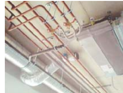
FIGURE 18. A ceiling mounted 4-pipe fan convector unit. Two or more supply ATDs can be connected to the unit. The supply air is blown out above the suspended ceiling and is then sucked into the fan convector together with the air inducted from the space below.
