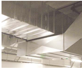
FIGURE 4. Cross-creased duct.
