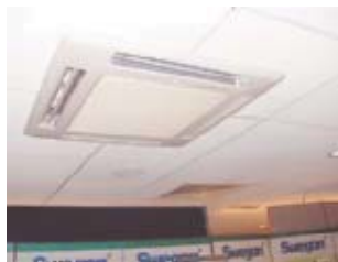
FIGURE 17. A fan convector designed as a ceiling cassette. The circulating air from the room is sucked in from directly beneath the unit and is discharged into the room, either cooled or heated, via the four supply air openings.
